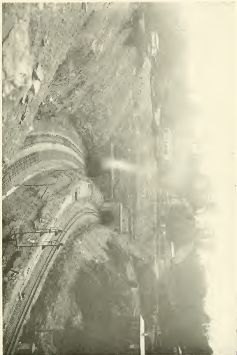
Kingwood Tunnel, showing three track tunnel system of the Baltimore and Ohio Railroad through Kingwood Mountain in Preston County, looking west from Tunnelton. The double-track tunnel to the left was completed May 27, 1912, at cost of approximately $1,500,000.
